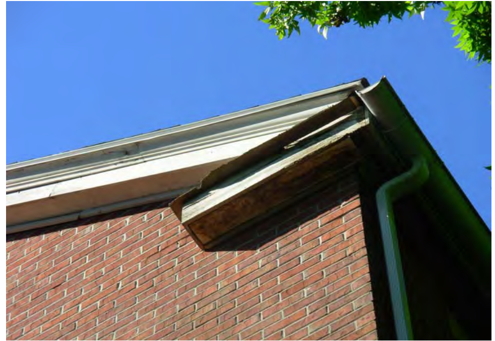
6. Wood deterioration, typical at soffits and trim
