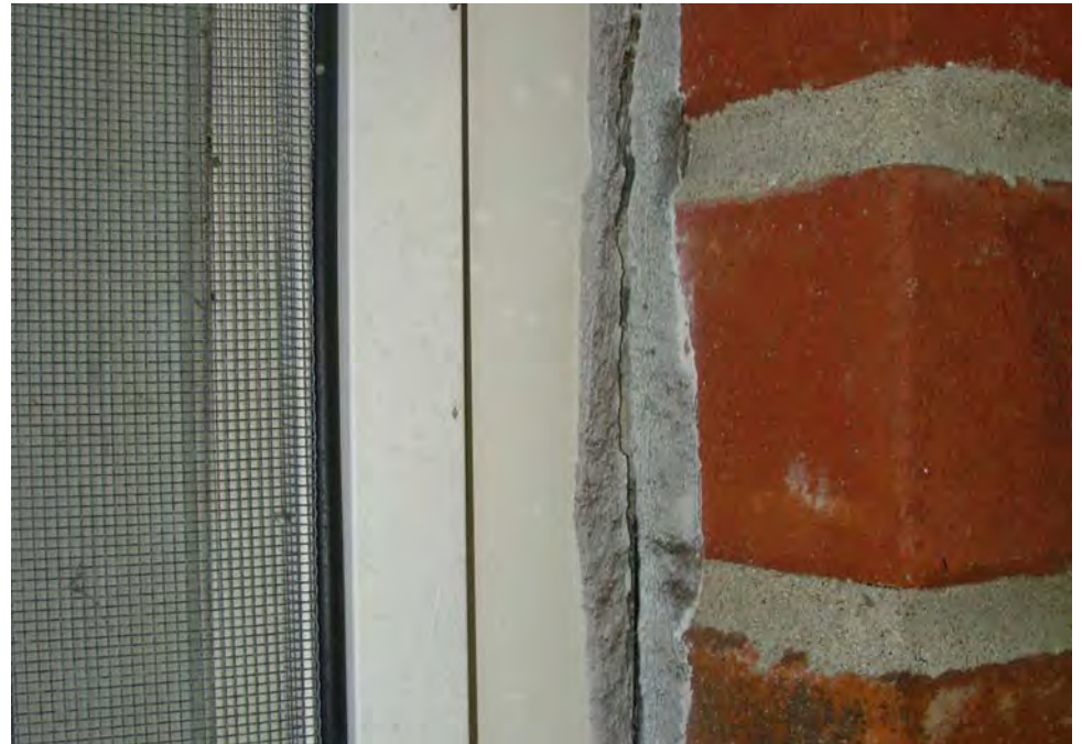
4. Caulking-sealant joint deterioration around windows
