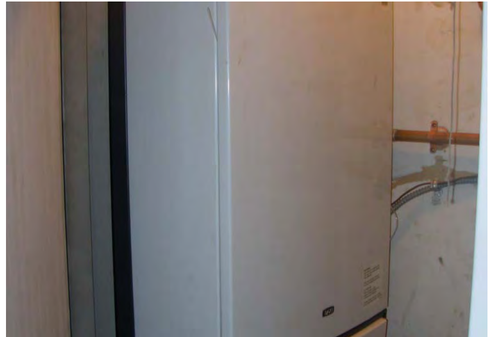
12. Wall pack heating and DHW generation equipment
