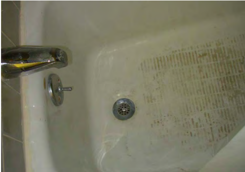
9. Unit tub finish deterioration, typical
