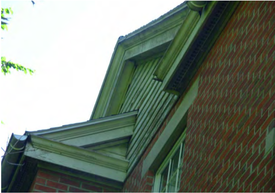
5. Soffit, fascia, gable siding deterioration - to replace
